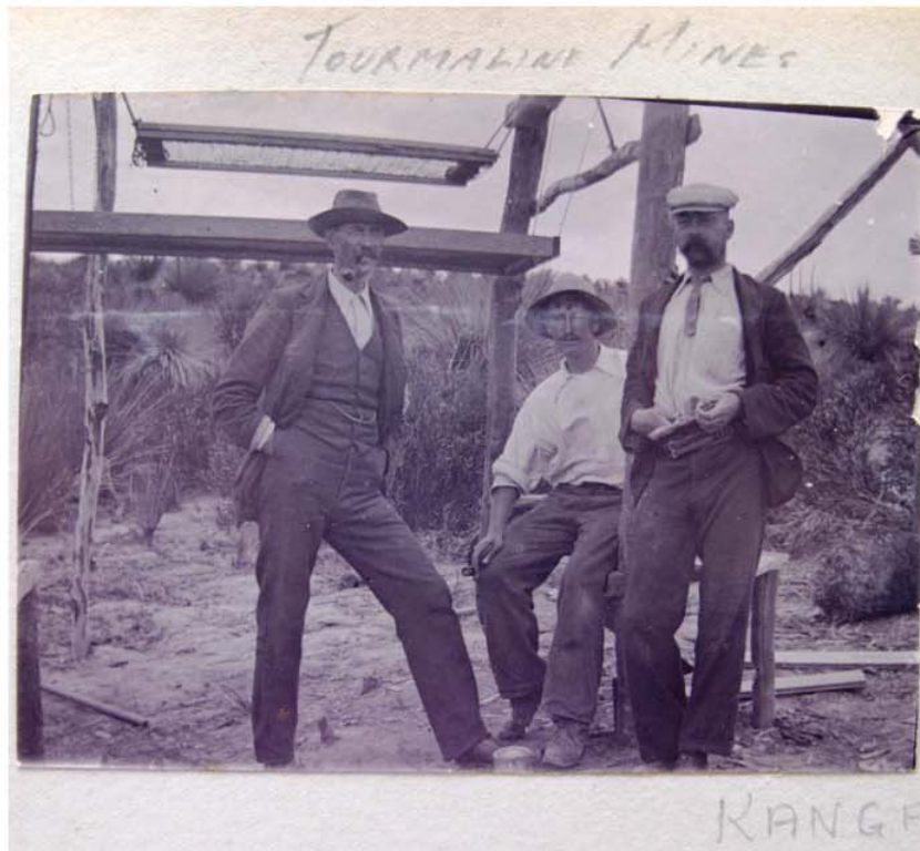
The jigger for sifting gems from their matrix at the tourmaline mine (JD Stow album, Penneshaw Maritime and Folk Museum).
