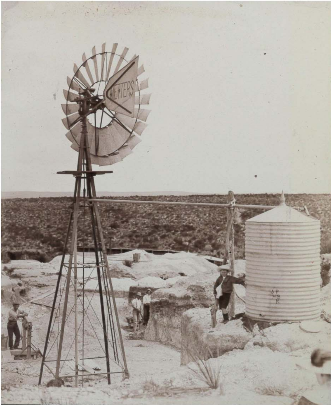
Open-cut mine and water pumping station, looking south. Fred Metters (1858-1937) began manufacturing water-pumping windmills at Adelaide with his 'Windmotor' in 1896. A shed runs behind on the perimeter. A few rail lines are laid. The woman in a hat in the lower right corner was no doubt a companion of the photographer. The tank is initialled JP/HB/K which John Radcliffe in a personal communication thinks with reason stands for John Provis, Hog Bay, Kangaroo Island (J.C. Radcliffe Collection)
