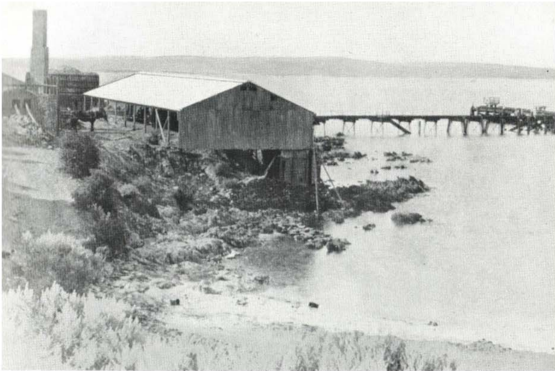
Penneshaw brickworks and jetty. View northwards. The mainland lies on the horizon. Probably 1908 (State Library of South Australia, B 50426). 'The works ... consist of a manager's office, engine house, two drying sheds (one 60 feet by 27 feet and the other 100 feet by 30 feet) a circular kiln which will hold about 23,000 bricks and a new kiln in course of erection which, when completed, will hold 35,000 bricks.' (Unohoo, 'Kangaroo Island China Stone and Clay Company', Kangaroo Island Courier , 3 October, 1908, p6a).
