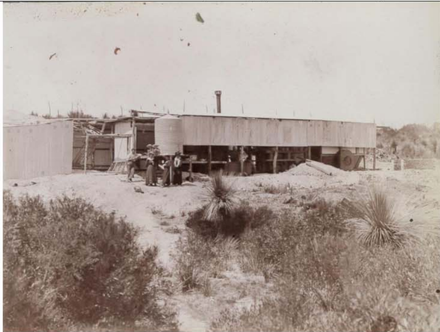
The china stone and clay mine. Water from the windmill was piped across into the machinery shed. Is it a basalt roller leaning against the shed, and an experimental brick wall, top right? The mine, at the lowest level of the basin-like grounds, gave gravitational access to trucks running from the diggings (J.C. Radcliffe Collection)
