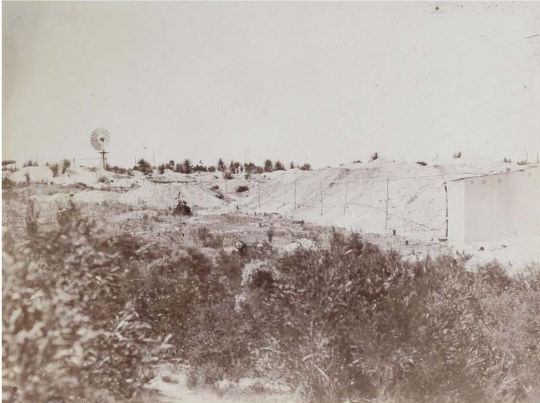
The thin water-pipe from the windmill to the shed is propped up on Y-shaped saplings along the front of the ore dumps; looking north. Both are difficult to distinguish (J.C. Radcliffe Collection)
